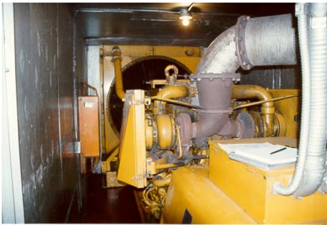
Photo 2 View of the 700 kW Portable Diesel #1 manufactured by Caterpillar.
