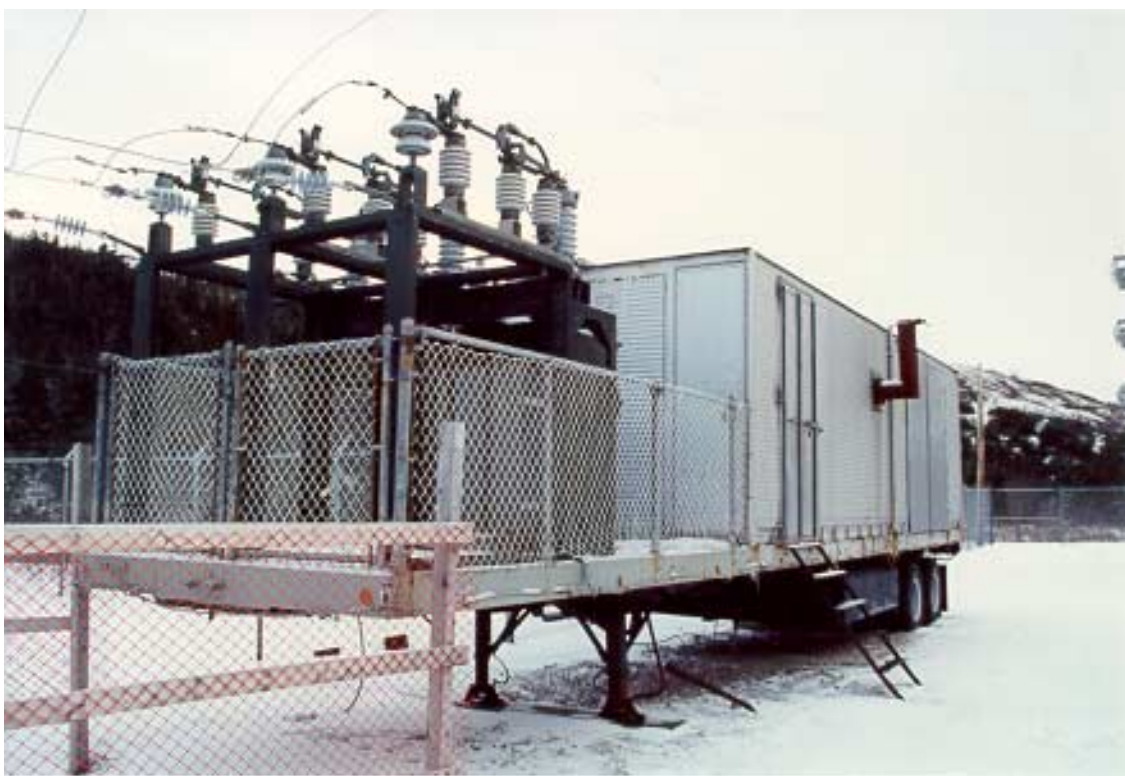
Photo 3 View of Portable Diesel #2 unit with trailer unit and transformer.
