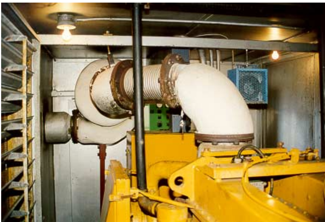
Photo 4 View of the 670 kW Portable Diesel #2 manufactured by Caterpillar.
